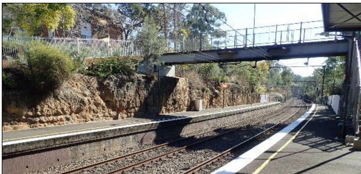
Figure 4.17 View from Platform 2 looking north-west at the sandstone railway cutting on Platform 1 and the Sedimentary Dykes in the vicinity of the footbridge.
