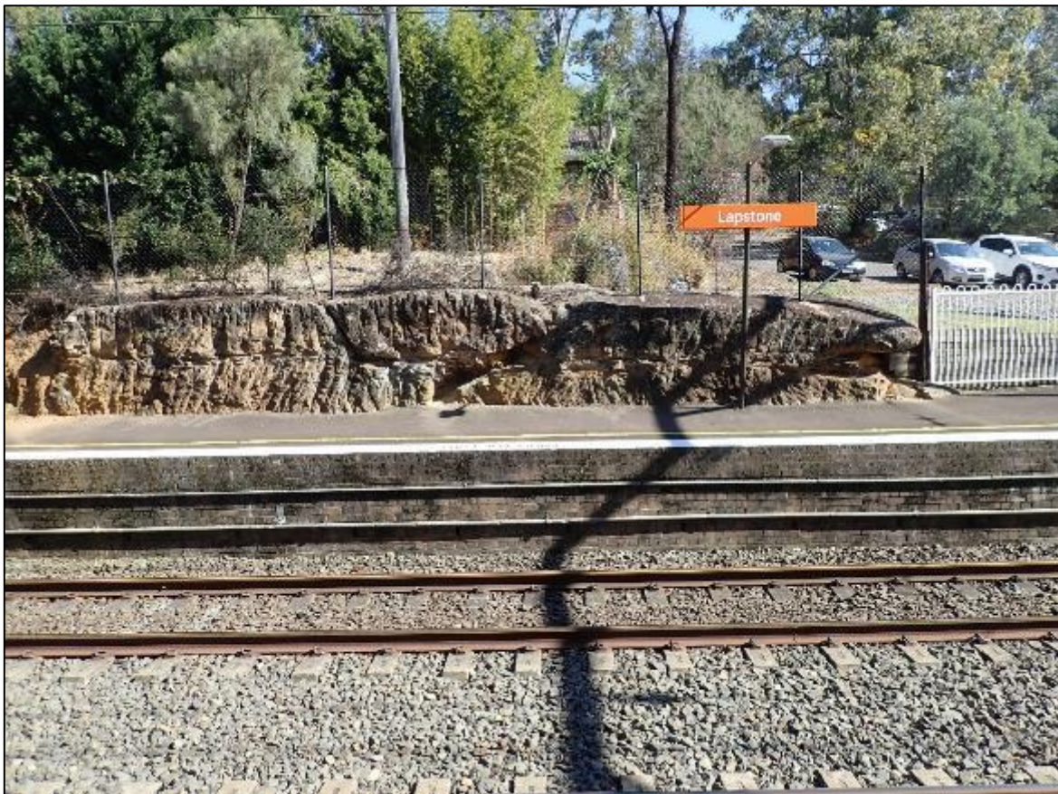
Figure 4.19 Eastern elevation of the sandstone railway cutting and sedimentary dykes south of the Lapstone Station building, south-east of the car park.
