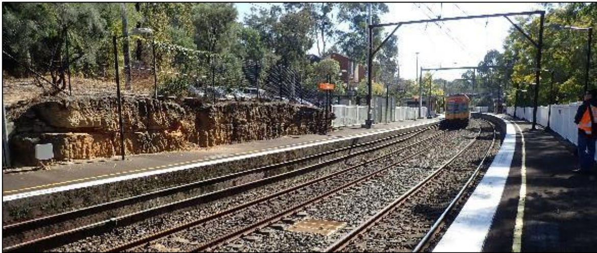
Figure 4.20 Eastern elevation of the sandstone cutting, showing the extent of the sedimentary dykes at the south end of Platform 1.
