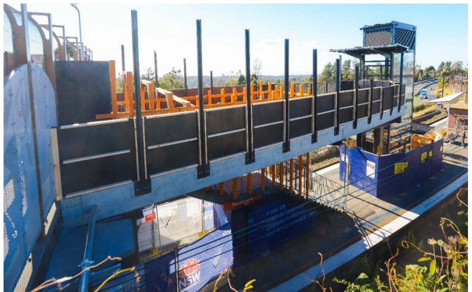
Photo of the new lift structure recently installed at Hazelbrook station. Over the next six months, this lift will be fitted and tested.
