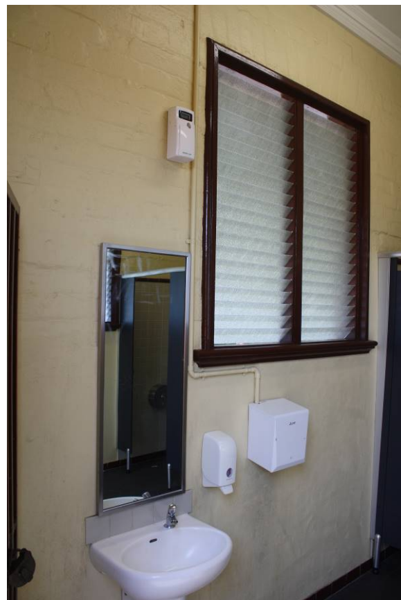
Plate 21 Detail of the current fixtures and fittings inside the male toilet. Note the original window and frosted glass.
