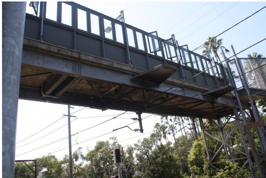
Plate 5 Detailed view of the underside of the footbridge. Showing the original subdeck structure associated with the footbridge, and the modern balustrades and windows.
