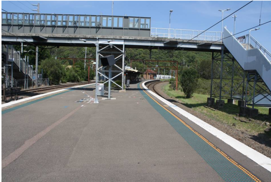
Plate 4 View of the western (Hawkesbury River) side of the footbridge at Hawkesbury River Station (view south), showing modified footbridge balustrades and anti-throw screens.
