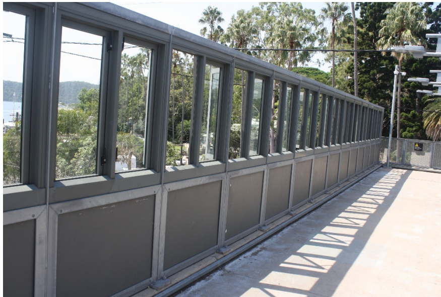
Plate 10 Detail view of the modern balustrade and operable windows on top of the footbridge.
