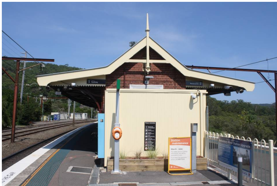
Plate 17 External view of the privacy screen currently installed in front of the entry to the male toilet.
