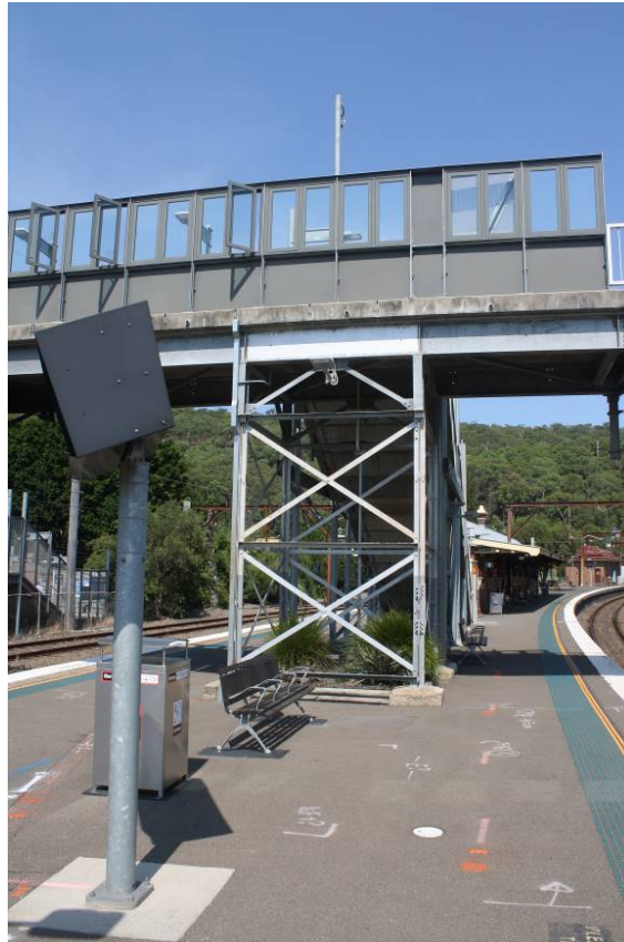
Plate 6 View of one of the box trestles supporting the footbridge (view southwest)
