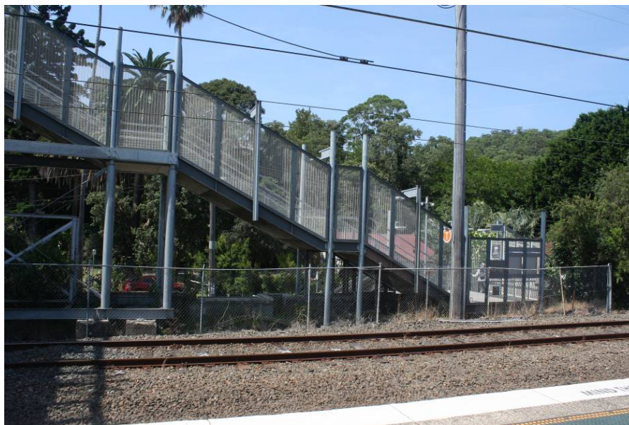
Plate 7 View of the new supports installed under the staircase leading from Dangar Road to the footbridge (view east).
