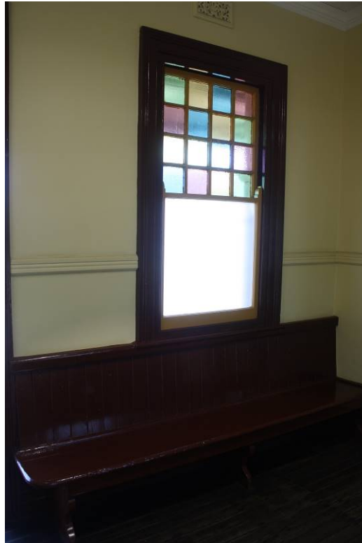
Plate 13 Detailed view of one of the sash windows, cathedral glass, dado rail and original bench seat.
