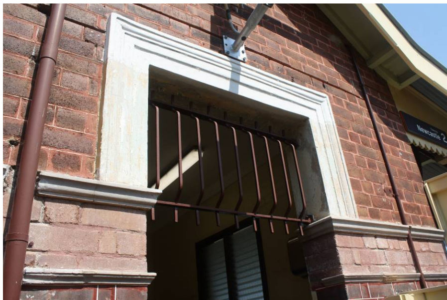
Plate 19 Detail of the metal grate installed where a transom window was previously.
