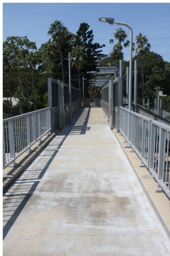
Plate 9 View from the top of the footbridge. Note the lower balustrade installed on the western half of the footbridge and modern concrete deck (view east)
