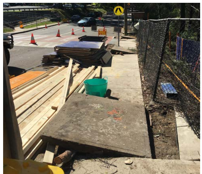
Image of Burfitt Parade mosaic removal in progress
