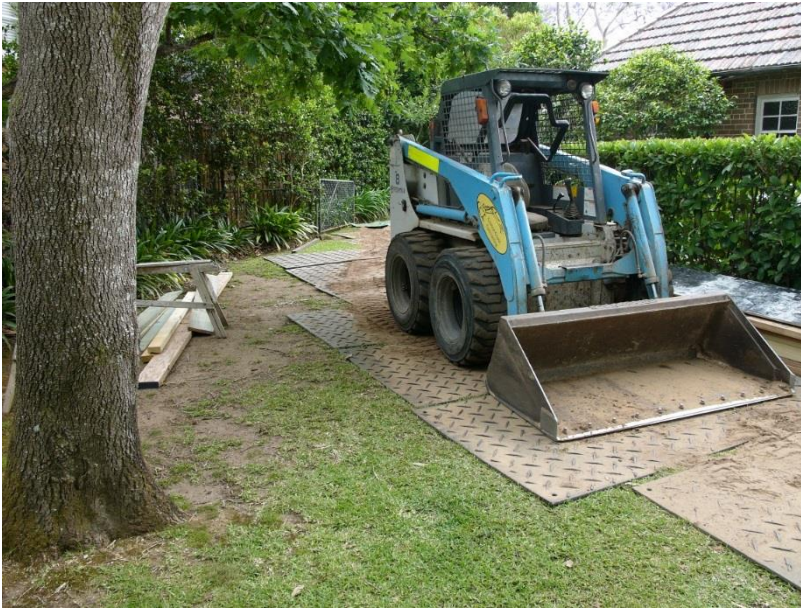
Figure 4 – Showing typical detail for truck mats.
