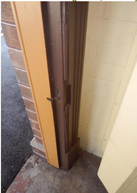
Figure 27: View of early door lock within existing door frame for storeroom. West aspect.
