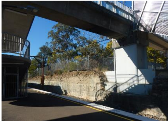
Figure 13: View of concrete plinth infill in rail cutting, northeast aspect.
