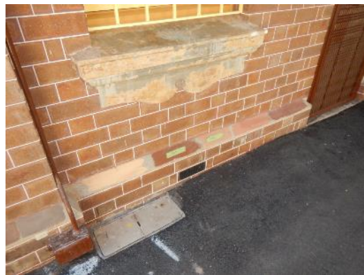
Figure 22: View of island platform building bricking, showing repointing, window lintels and recently painted brickwork. West aspect.
