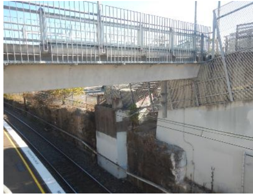
Figure 16: View of pedestrian footbridge with steel balustrade and glass inserts. Note the remnant original concrete plinth fabric. Southwest aspect.
