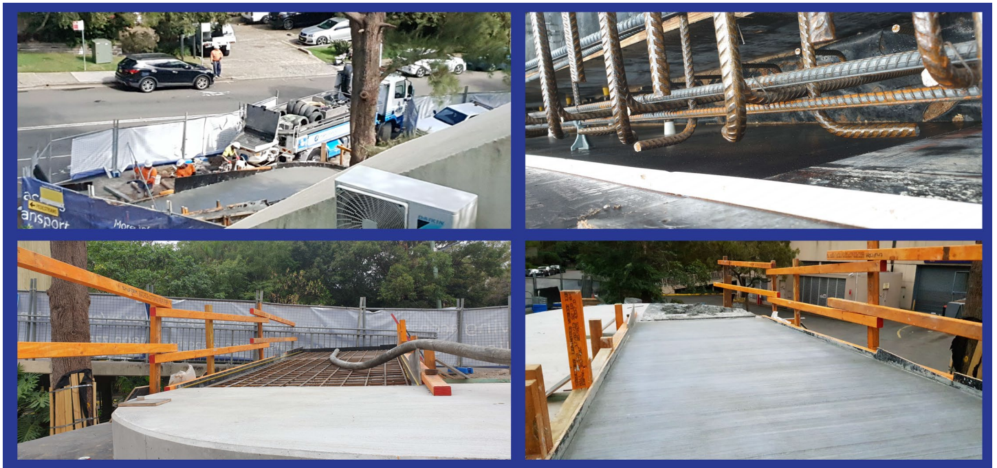
Image: Construction updates of new ramp
