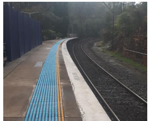
Photo of the upgraded tactile indicators at Glenbrook Station
