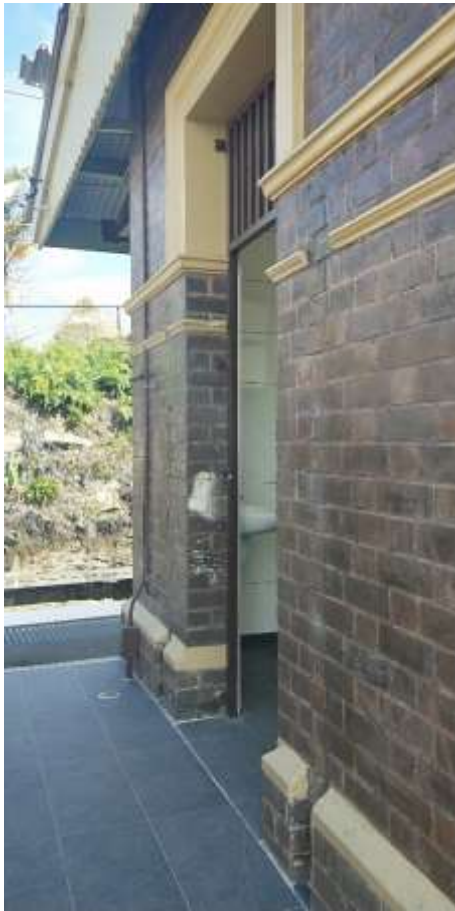
Figure 18. Entrance to male toilets showing brickwork needing repointing (Source: Extent)
