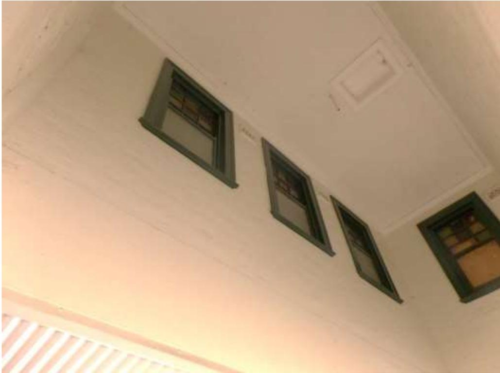
Figure 15. Interior of the pavilion, west side showing the original windows remaining behind exterior boarding
