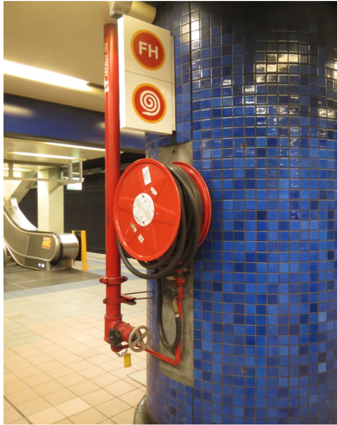
Figure 10 Decorative blue tile removed for installation of fire hose
