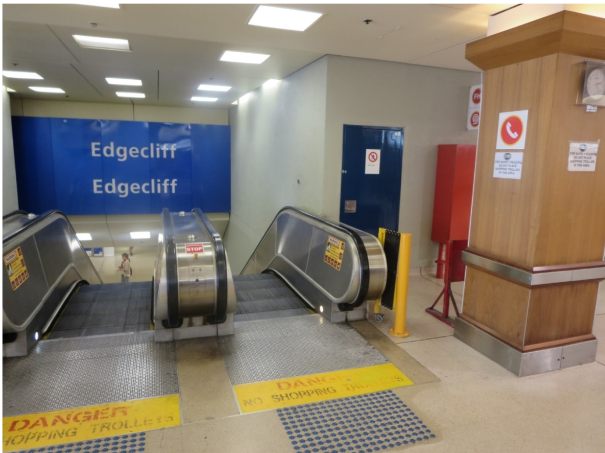
Figure 6 Edgecliff gallery showing original terrazzo floors and replacement columns and ceiling
