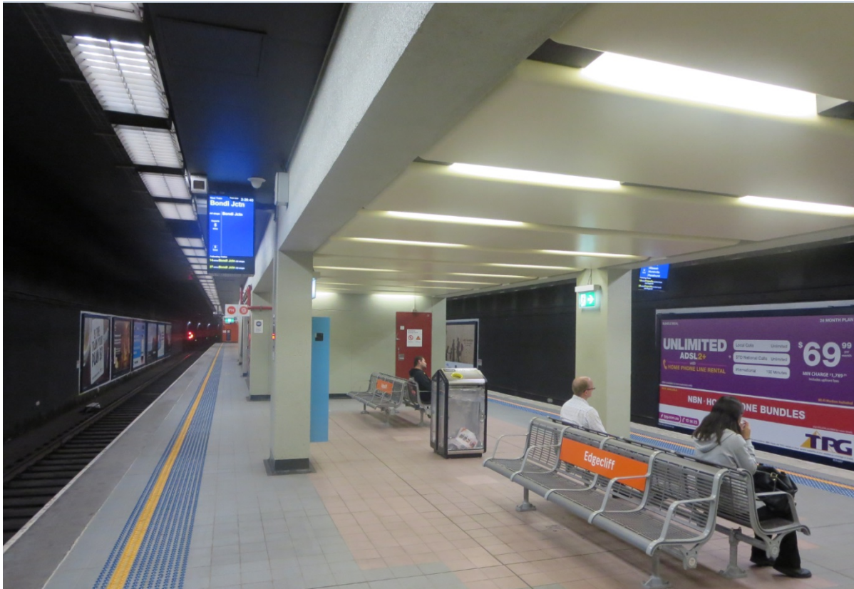
Figure 8 Platform at Edgecliff Railway Station, showing moulded plywood ceiling, tile floors and aggregate render walls
