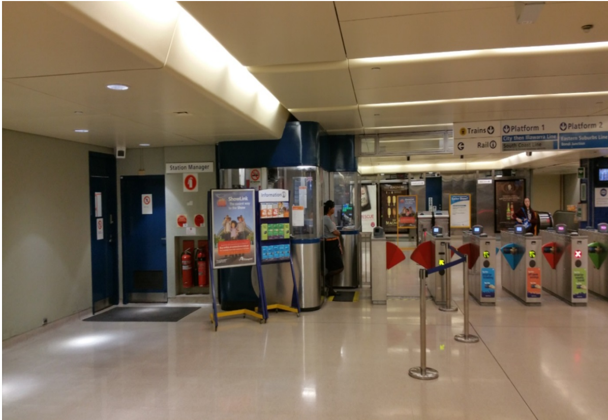
Figure 7 Concourse at Edgecliff Railway Station, showing moulded plywood ceiling, terrazzo floors, aggregate render walls, and stainless steel cladding
