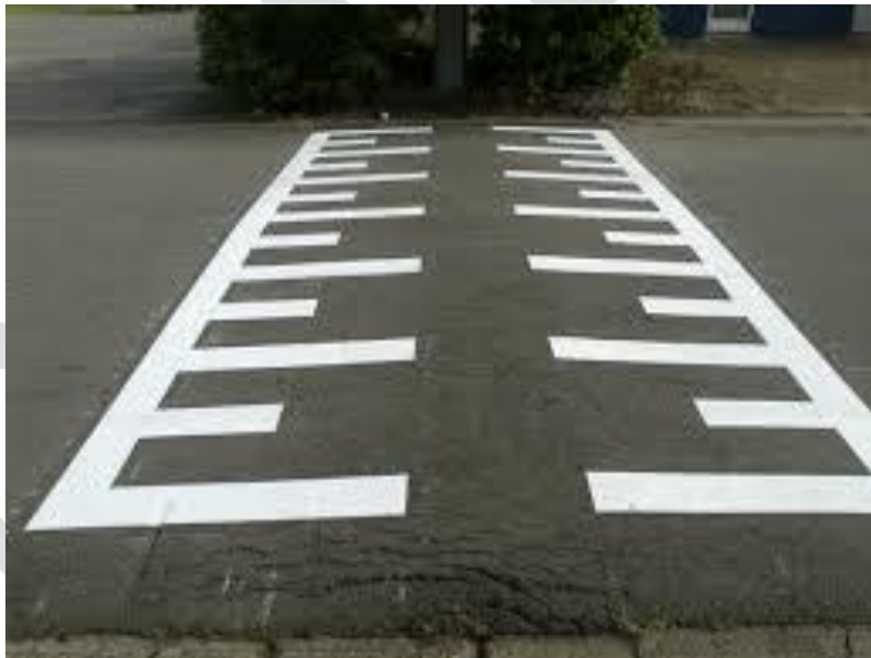
Figure 3-1 Example of piano keys road markings (Source: safetyfirstlinemarking.com.au )
