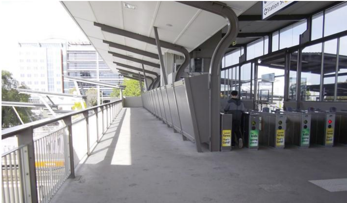
Figure 2.16: View of Existing Penrith Station Overhead Concourse
