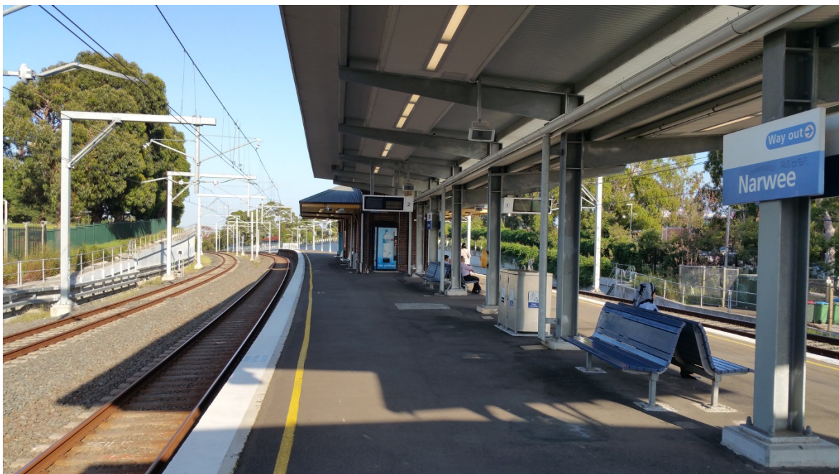
Figure 7 View looking west on the 1931 platform of Narwee Station which is listed under s.170 of the Heritage Act 1977 (NSW)
