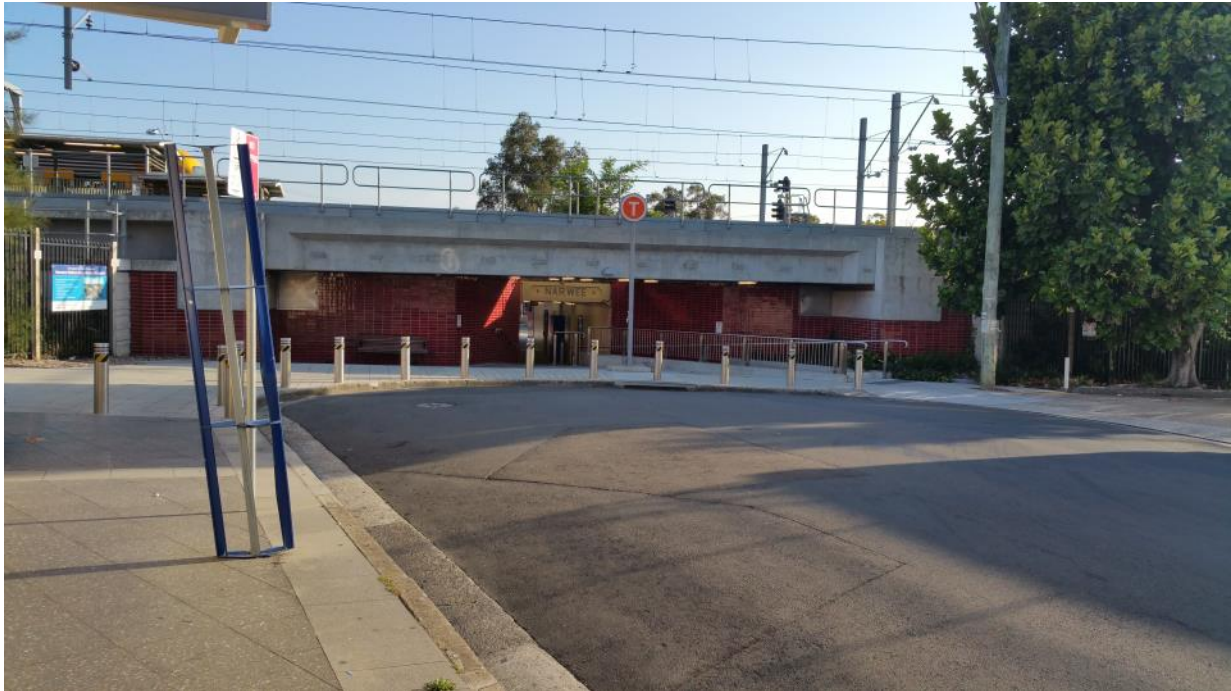
Figure 4 View towards Narwee Station from Hurst Place pedestrian underpass entrance
