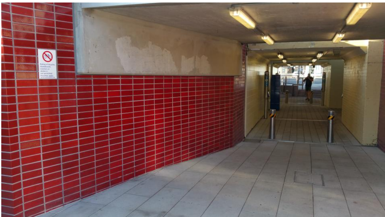
Figure 5 View towards Narwee Station from Hannans Road pedestrian underpass entrance
