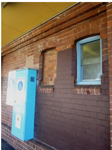
Figure 20 Bricked-in window opening and painted brickwork, south facade (AECOM, 2016)
