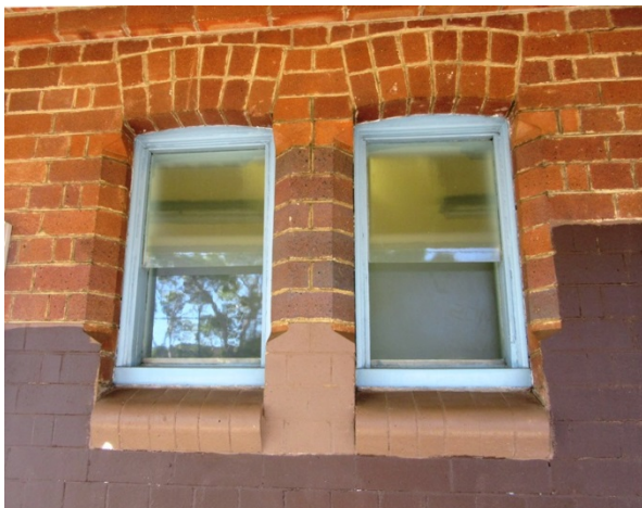
Figure 18 Original windows to men's bathroom, bullnose sills and chamfered brickwork (AECOM, 2016)
