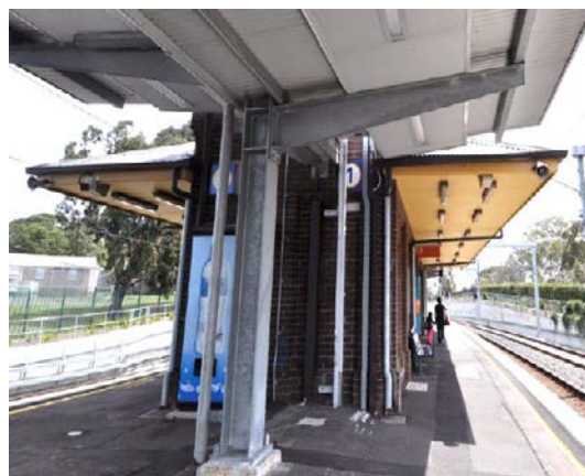
Figure 9 Current status of east elevation platform. Note obstructed view of façade due to canopy, and placement of vending machine and service conduits and downpipes. (Rappoport, 2014a:10)
