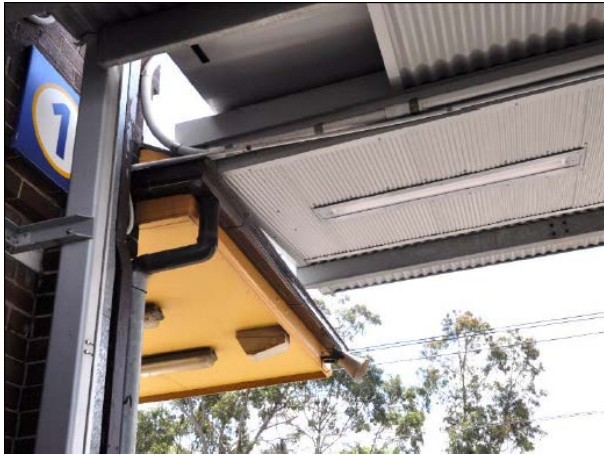
Figure 34 East façade of Platform Building showing poor junction with canopy roof, obstruction by canopy structure. (Rappoport 2014a: 12)
