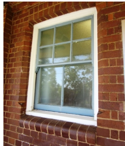
Figure 19 An original 6-pane upper sash window to north façade (AECOM, 2016)
