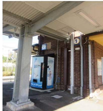
Figure 17 Platform Building, east façade showing intrusive attached conduit boxes and downpipes (AECOM, 2016)
