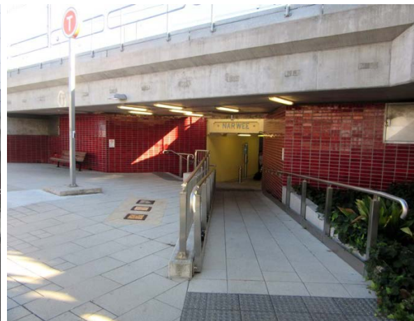
Figure 37 Non-DDA compliant ramp at southern entrance to station (AECOM, 2016)
