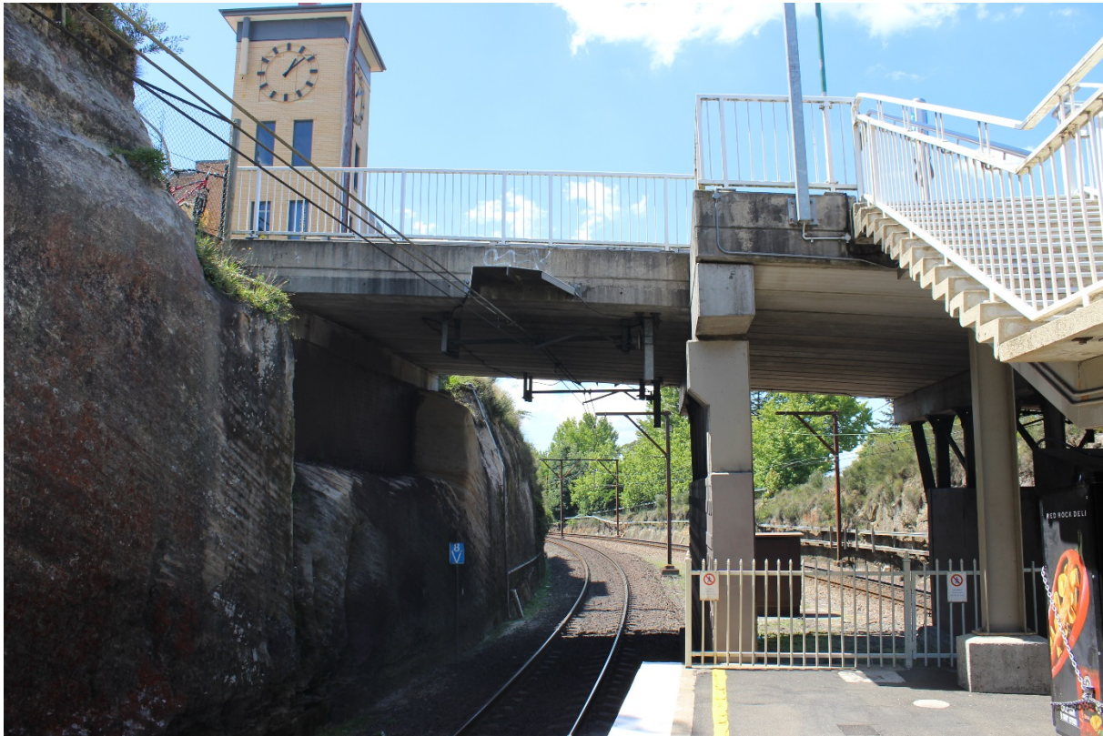
Figure 33: View of northern half of overbridge showing cut into sandstone embankment for the road surface. East aspect
