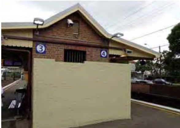
Heritage building on Platforms 3/4, looking east. The curtain wall around the old toilet facilities would be demolished and a new family accessible toilet would be provided.
