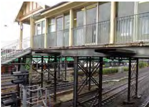
The trestle structure supporting the overhead booking office.
